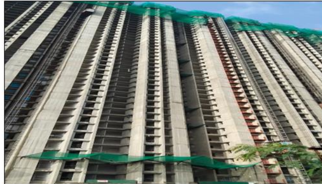
TOWER - 2 : 42nd slab ready to cast
