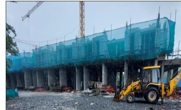
TOWER - 6 : 2nd slab WIP
