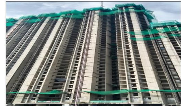
TOWER - 3 : 42nd slab ready to cast
