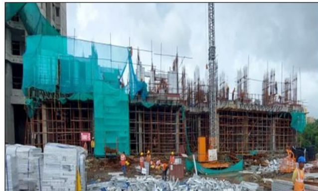
TOWER - 5 : 2nd slab WIP
