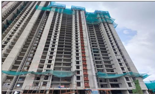
TOWER - 4 : 30th slab WIP
