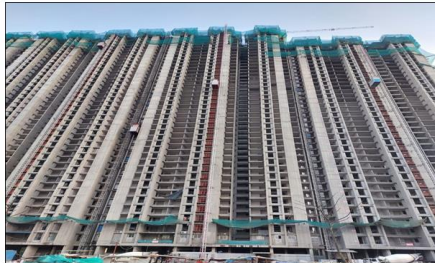
TOWER - 3 : Above Terrace works in progress
