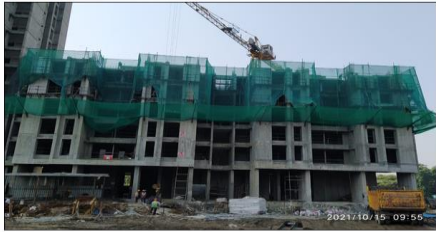
TOWER - 5 : 6th slab casting in progress
