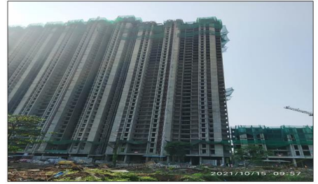
TOWER - 4 : 41st slab WIP
