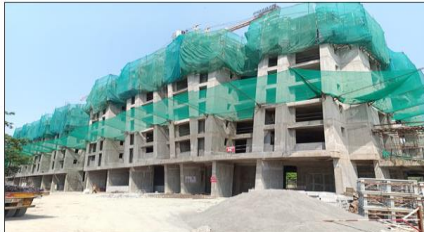
TOWER - 6 : 9th slab work in progress
