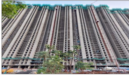
TOWER - 2 : Above Terrace works in progress
