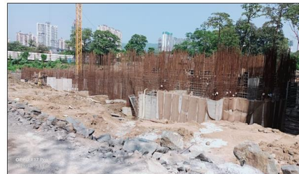
TOWER - 10 : Tie beam work in progress
