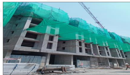
TOWER - 7 : 8th slab work in progress
