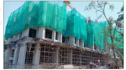
TOWER - 8 : 5th slab casting in progress
