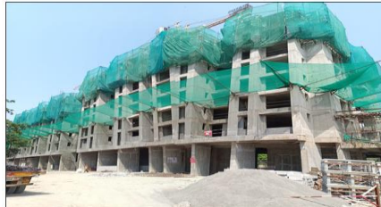
TOWER - 6 : 9th slab work in progress
