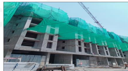
TOWER - 7 : 8th slab work in progress
