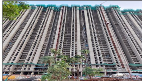
TOWER - 2 : Above Terrace works in progress
