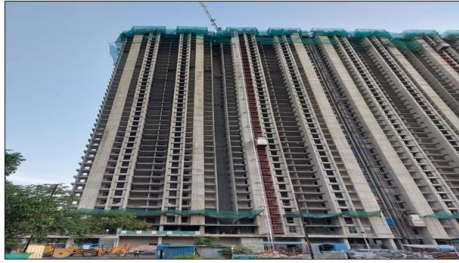
TOWER - 1 : Above Terrace works in progress
