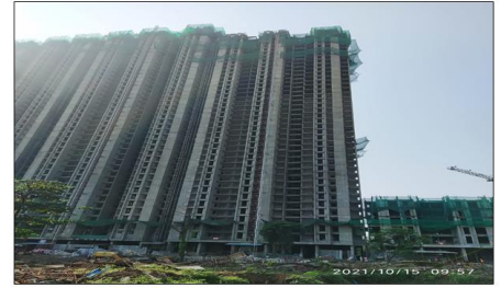
TOWER - 4 : 41st slab WIP
