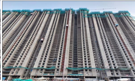
TOWER - 3 : Above Terrace works in progress
