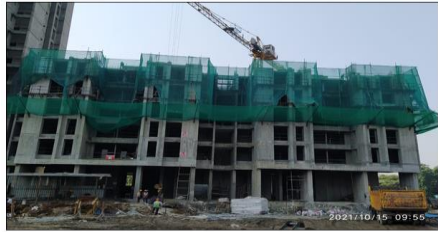
TOWER - 5 : 6th slab casting in progress
