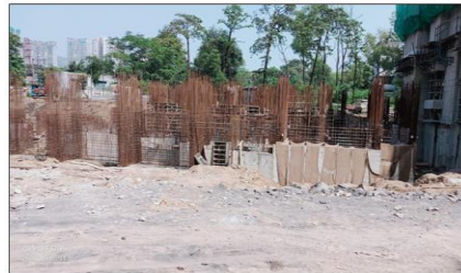
TOWER - 9 : Verticals above Tie beams upto Plinth in progress
