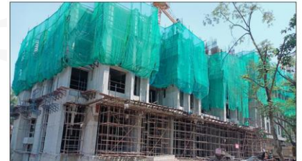
TOWER - 8 : 5th slab casting in progress
