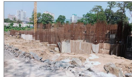
TOWER - 10 : Tie beam work in progress
