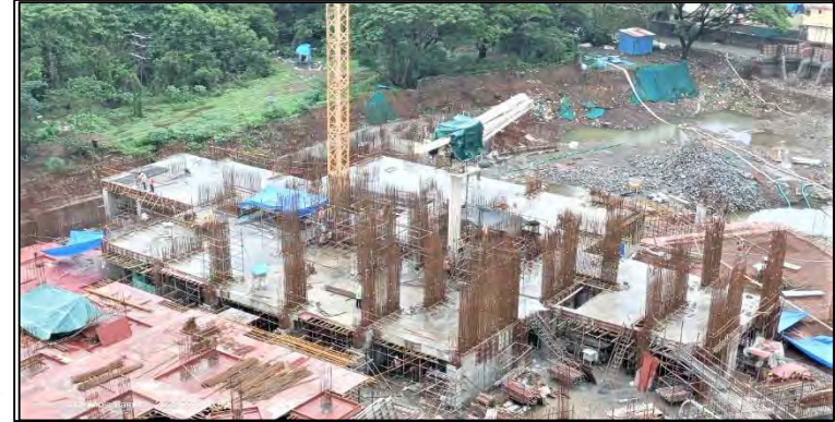
Tower B – Basement Slab & Foundation Work in Progress
