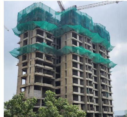
Tower (B) 10 th Floor Slab Completed
