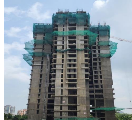
Tower (A) 18 th Floor Slab Completed
